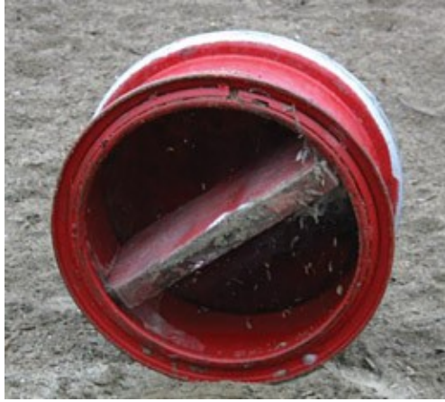
Underside of Pedestal
