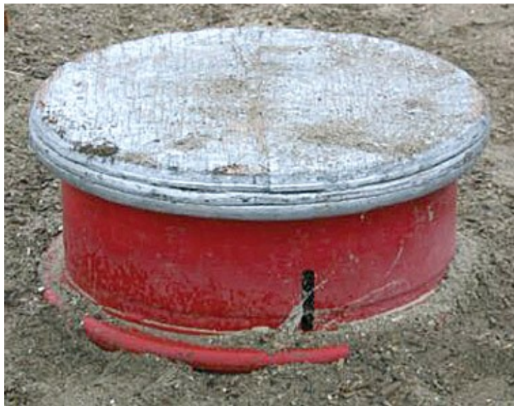
Top of Pedestal
